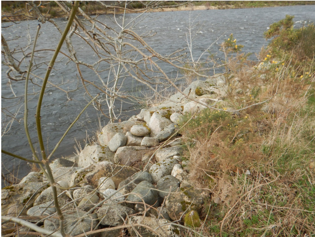
Plate 19: Exposed cobbles/boulders on river side of embankment at 14 th Tee
