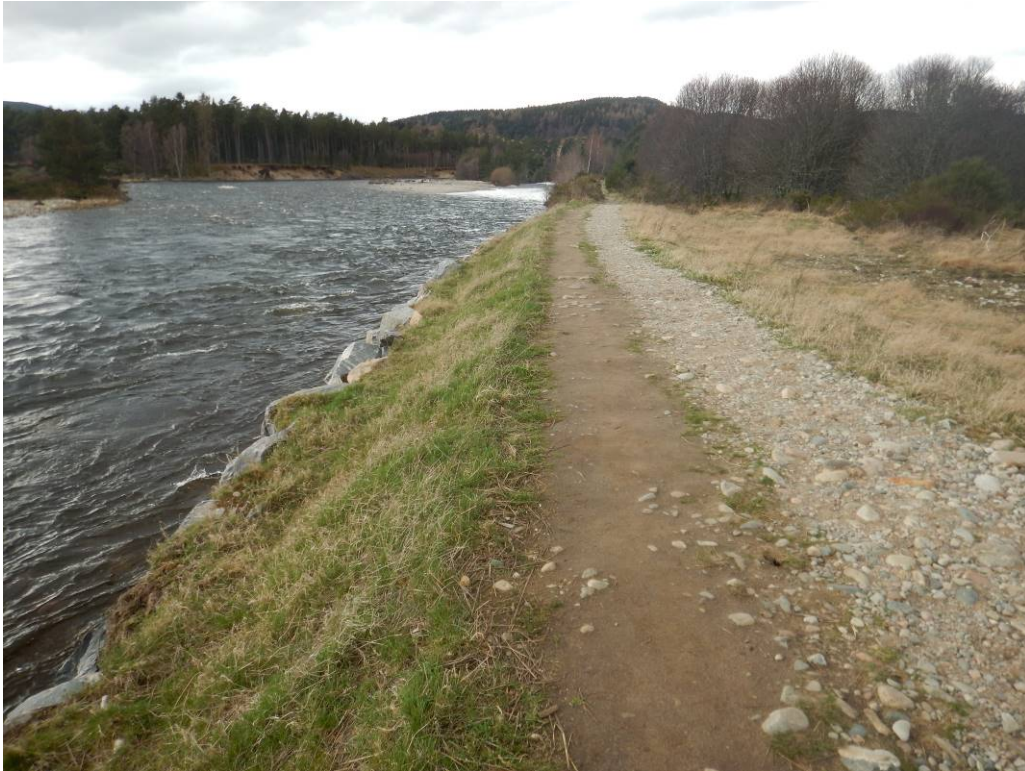
Plate 5: River side embankment with boulder toe
