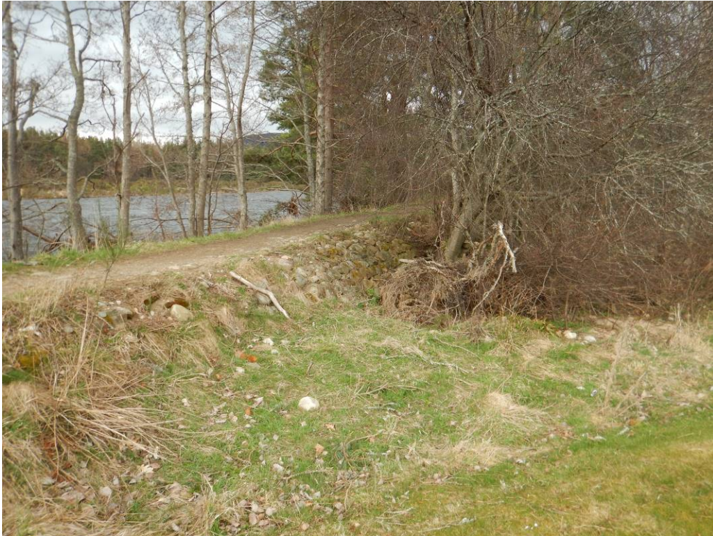
Plate 20: Masonry revetment to rear face of embankment north of 14 th Tee
