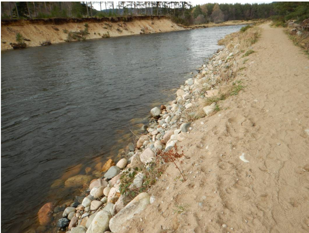
Plate 13: Un-vegetated face of re-profiled embankment
