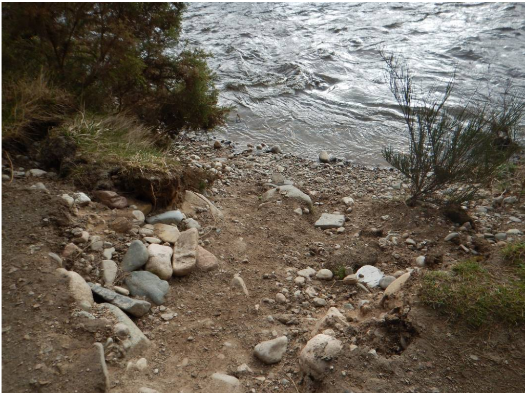
Plate 9: Partial breach of embankment at 36133,95261
