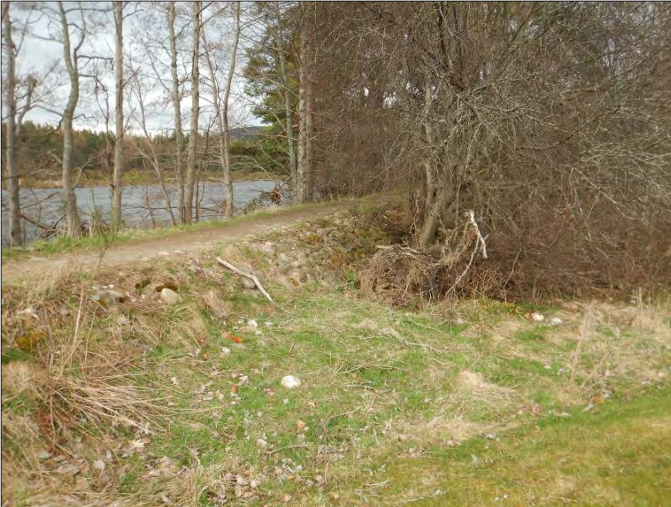
Plate 42 Masonry revetment to rear face of embankment north of 14th Tee (2018)
