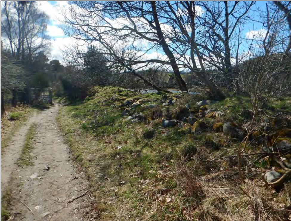
Plate 48 Typical view of embankment north of 36020,95756 (2018)
