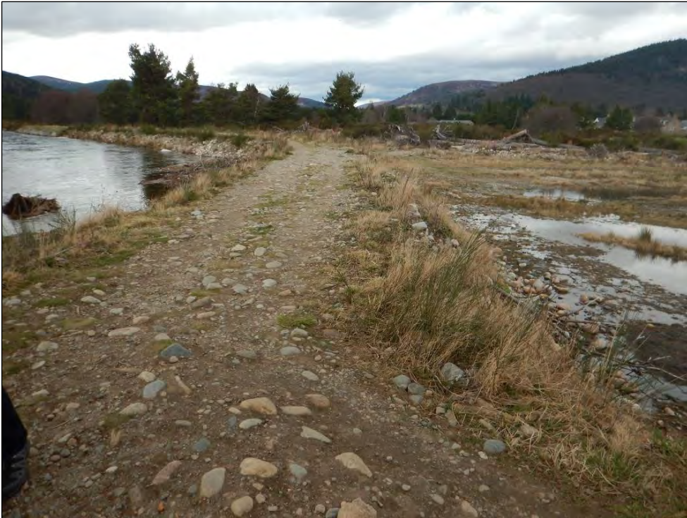
Plate 7 Embankment at south end of Golf Course looking NW (2018)
