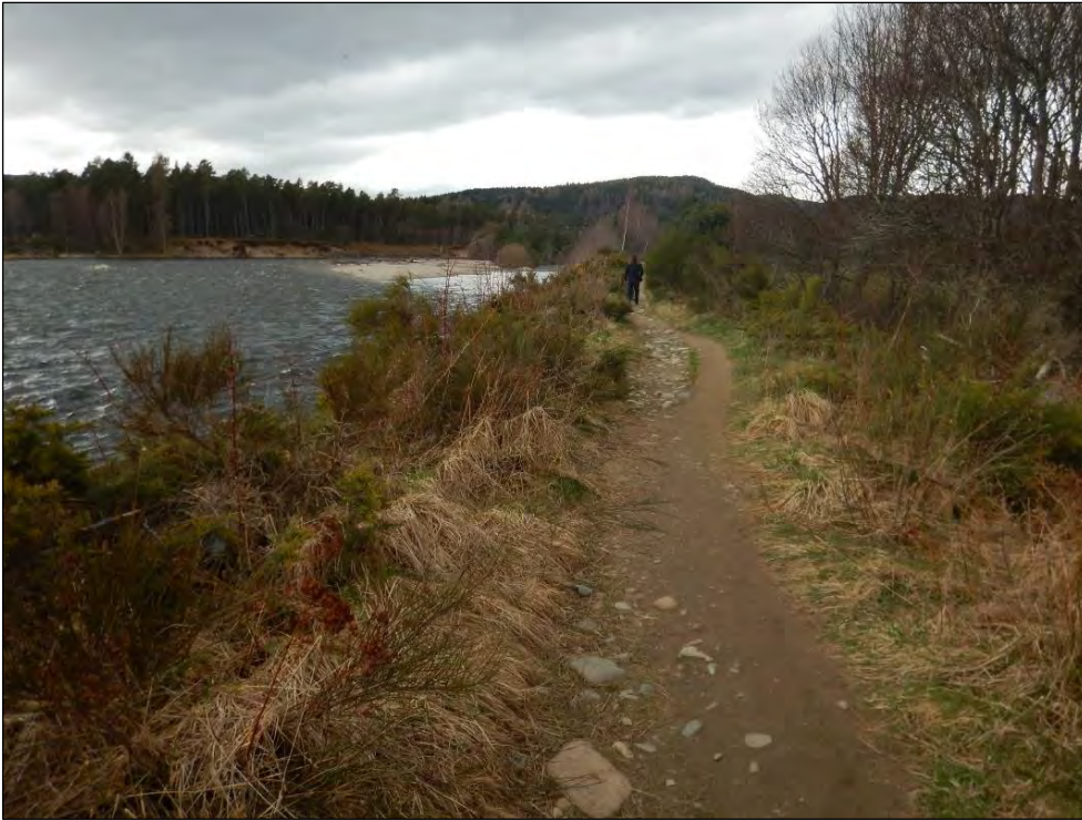
Plate 14 Vegetation on northern section of embankment with boulder toe (2018)
