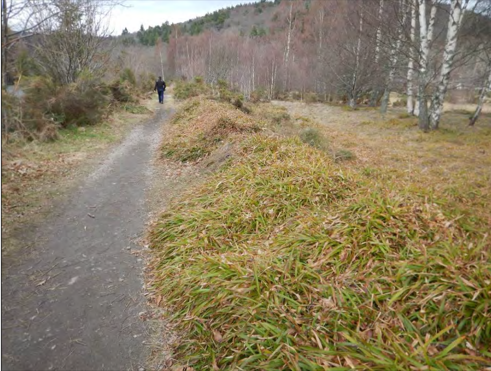
Plate 52 Low embankment on landward side of path (2018)
