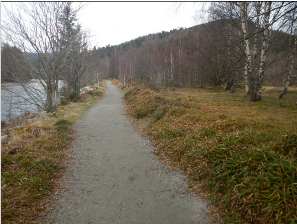
Plate 53 Low embankment on landward side of path (2022)
