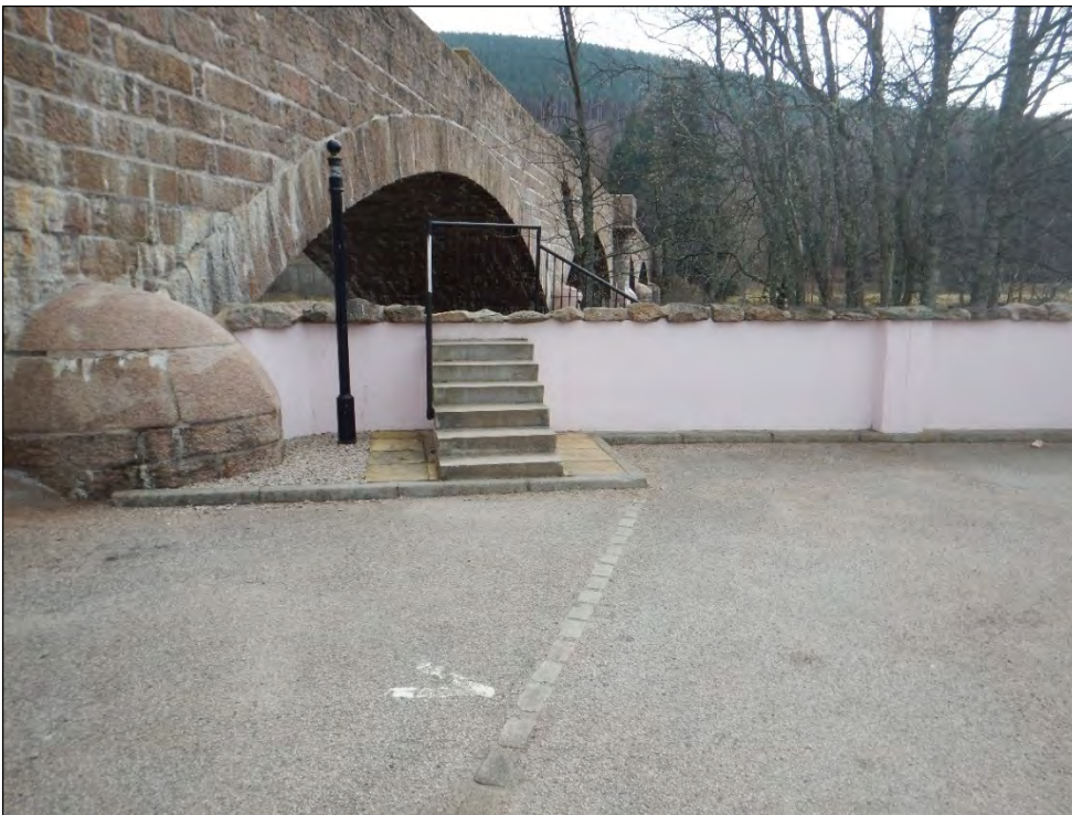
Plate 1 View of rear face of wall at Cornelian Square (2022)
