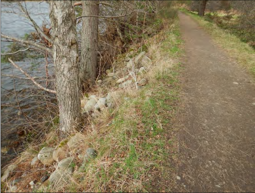
Plate 44 River face of embankment north of 14th Tee (2018)
