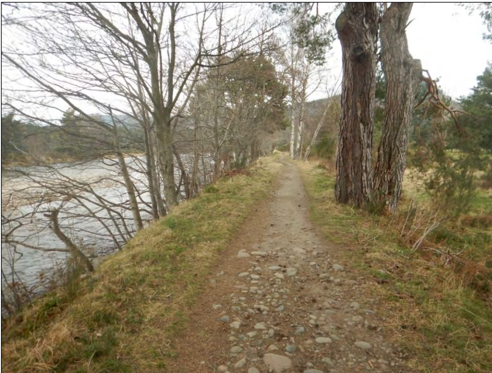
Plate 33 Typical view of embankment south of the 14th Tee (2022)
