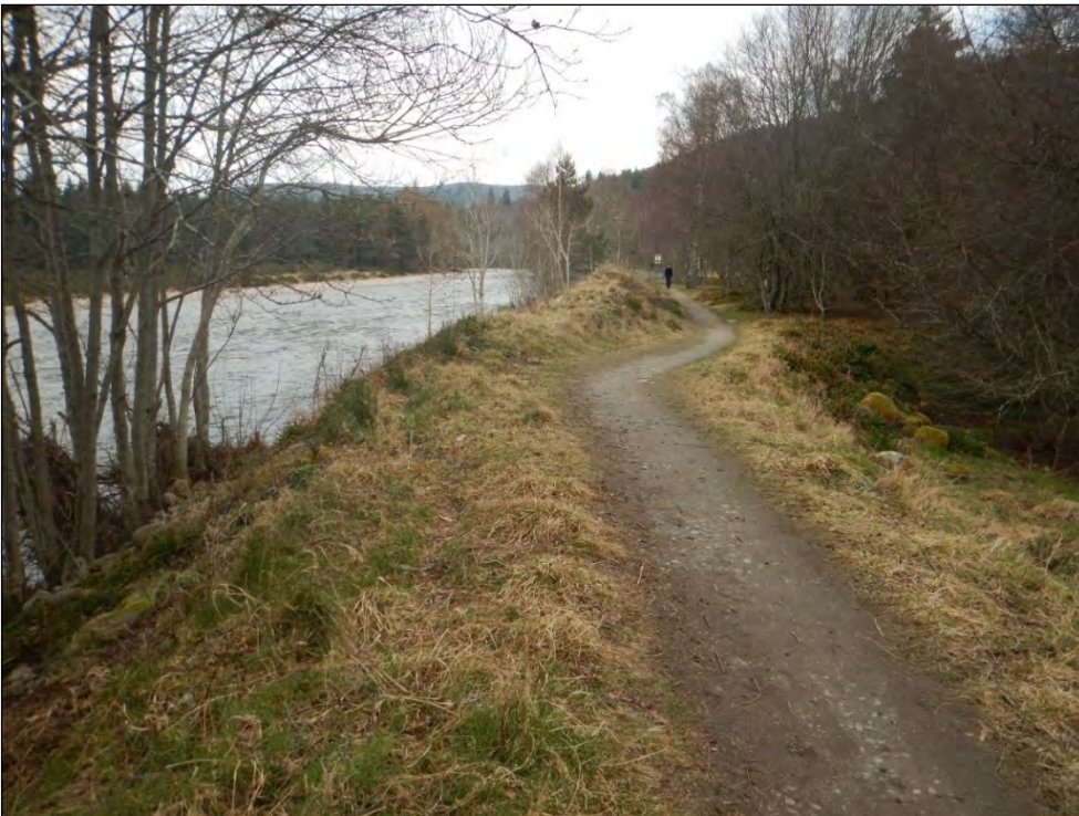
Plate 47 Transition of riverside path from top of embankment to land behind (2022)
