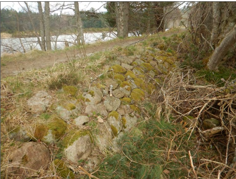
Plate 43 Masonry revetment to rear face of embankment north of 14th Tee (2022)
