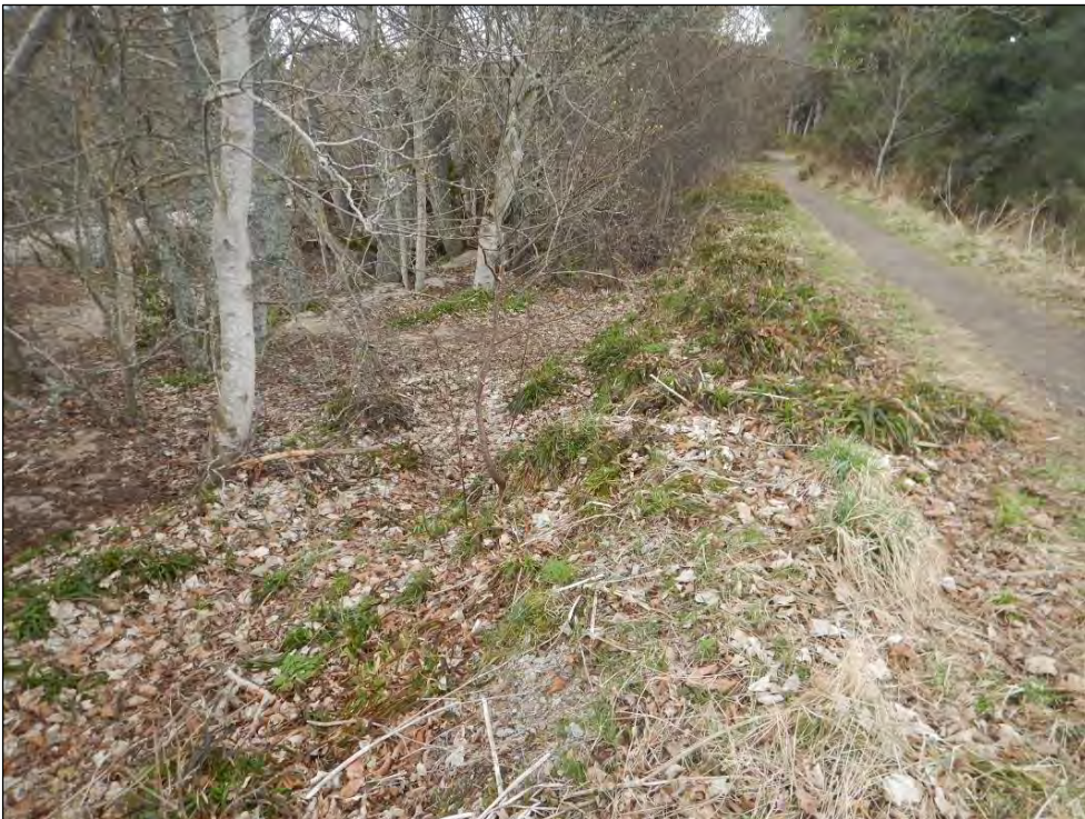
Plate 18 Typical view of embankment (2018)
