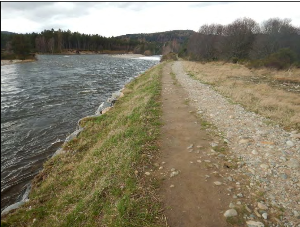
Plate 13 Embankment with boulder toe (2018)
