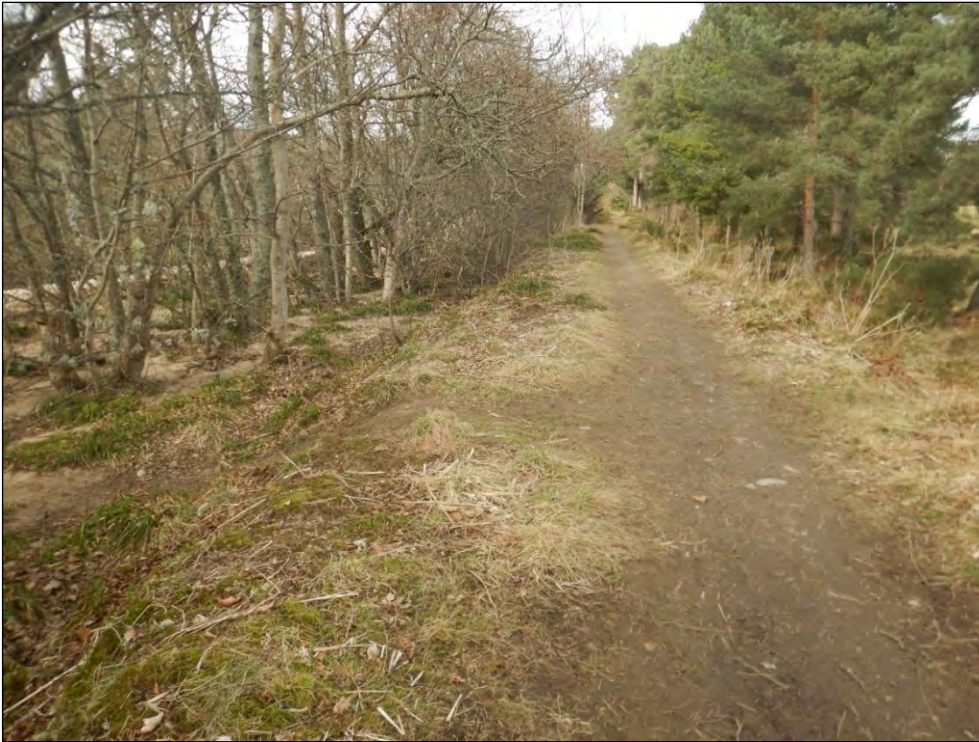
Plate 21 Typical view of embankment (2022)
