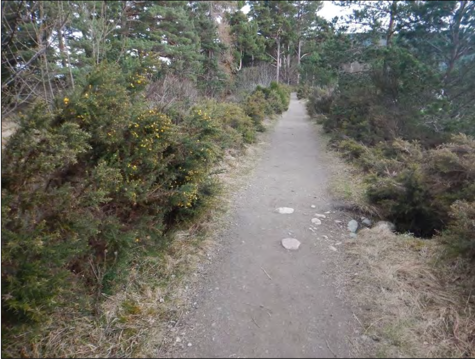
Plate 23 Pathway on embankment crest (2018)
