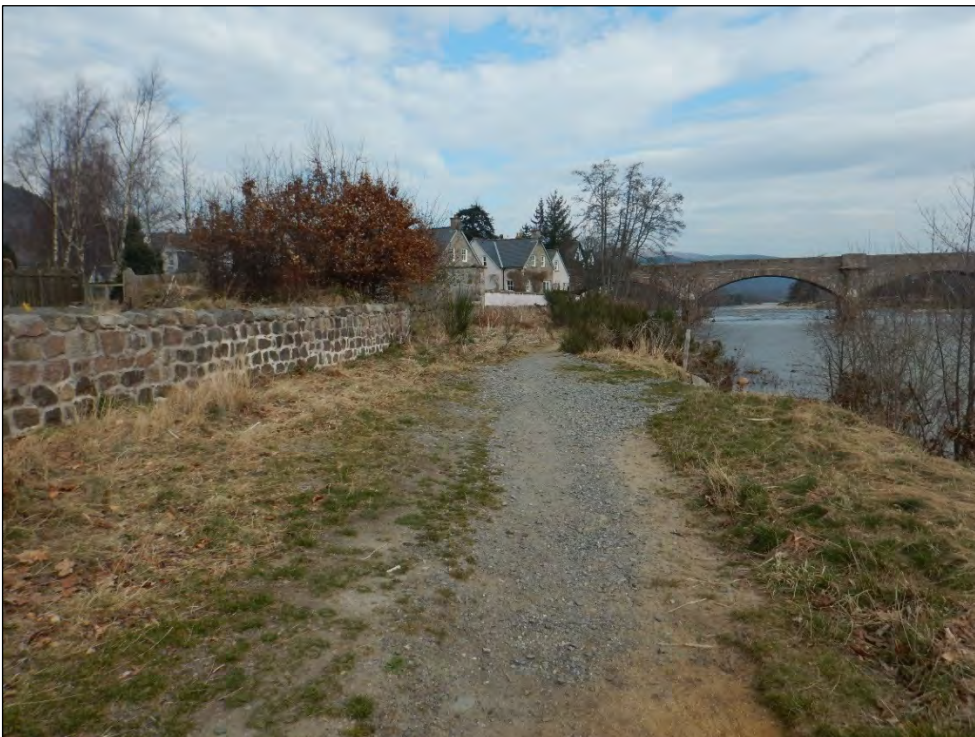
Plate 3 Overview of walls upstream of Royal Bridge (2022)
