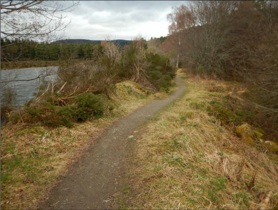
Plate 46 Transition of riverside path from top of embankment to land behind (2018)
