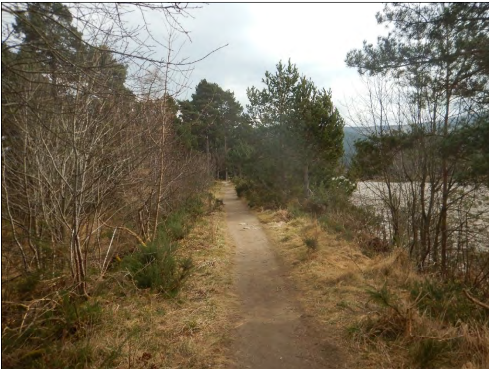
Plate 24 Pathway on embankment crest (2022)
