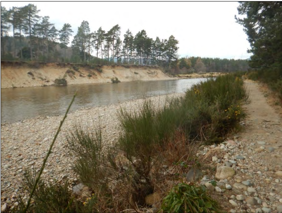
Plate 30 Former unvegetated face of embankment (2022)
