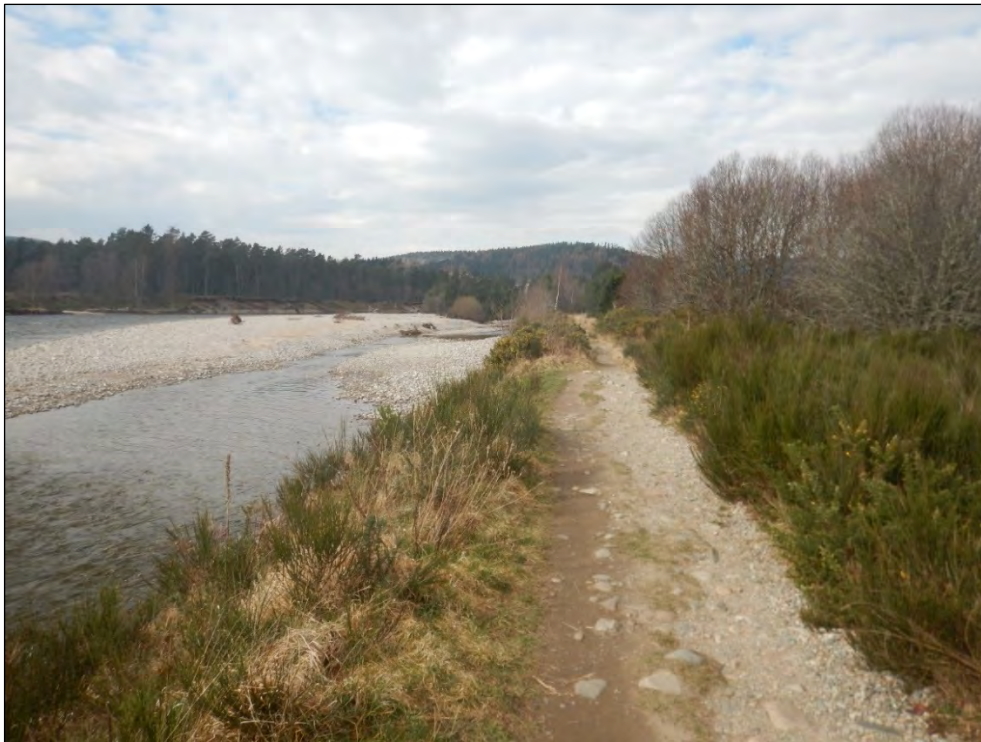
Plate 16 Vegetation on northern section of embankment with boulder toe (2022)
