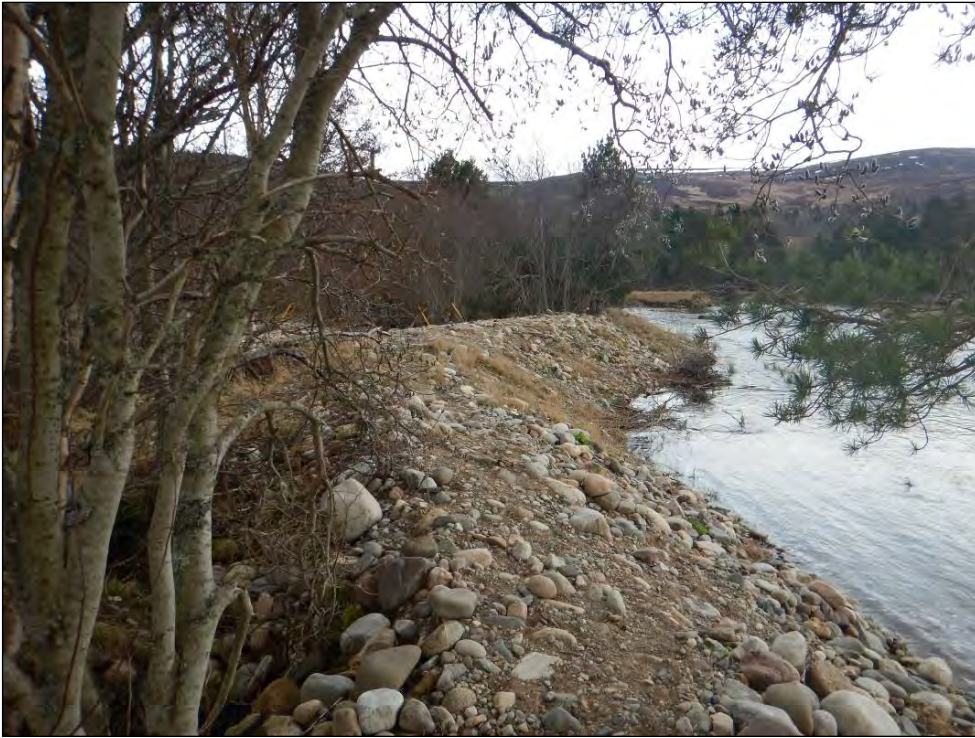
Plate 9 Embankment at south end of Golf Course looking SE (2018)
