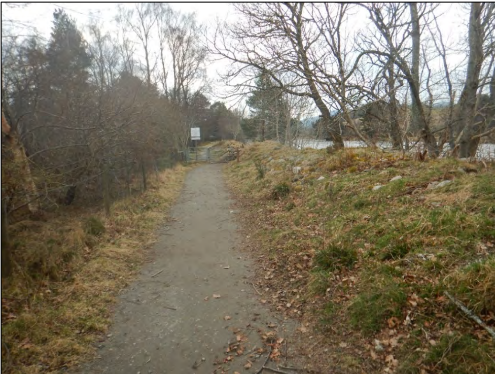
Plate 49 Typical view of embankment north of 36020,95756 (2022)
