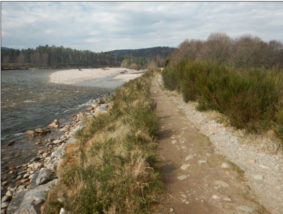
Plate 15 Embankment with boulder toe (2022)
