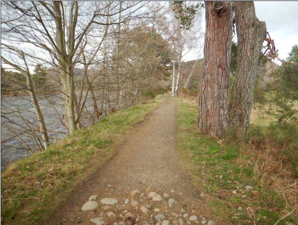
Plate 32 Typical view of embankment south of the 14th Tee (2018)
