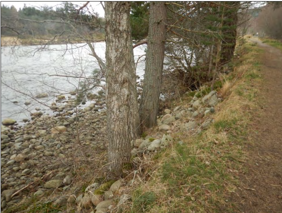
Plate 45 River face of embankment north of 14th Tee (2022)
