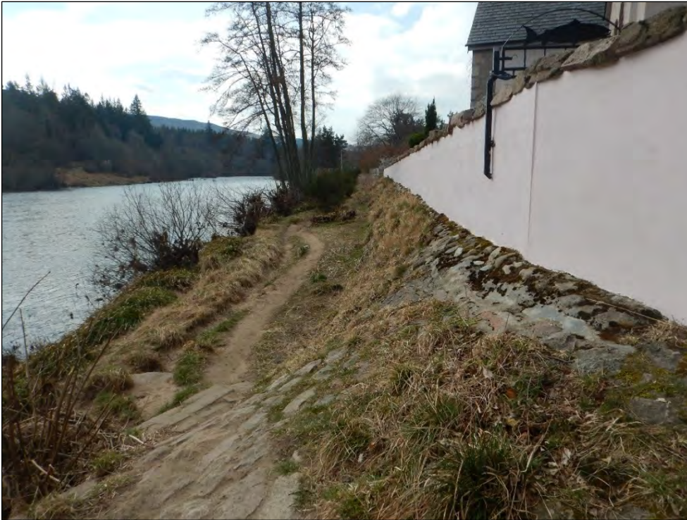
Plate 2 View of riverside face of wall at Cornellian Square (2022)
