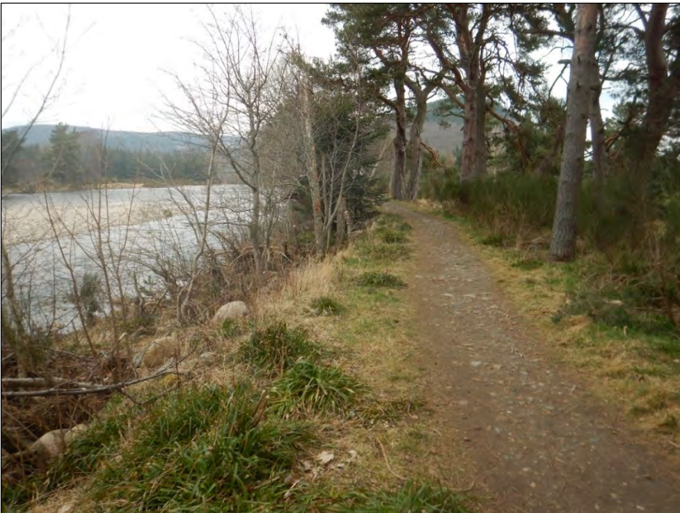
Plate 35 Embankment south of the 14th Tee showing more vegetation over exposed cobble (2022)
