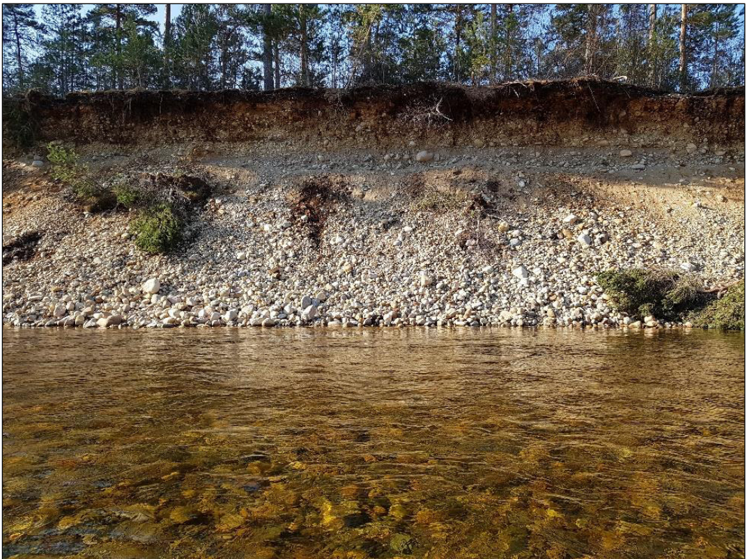
FIGURE 4 – FLOOD BANK ON RIGHT BANK
