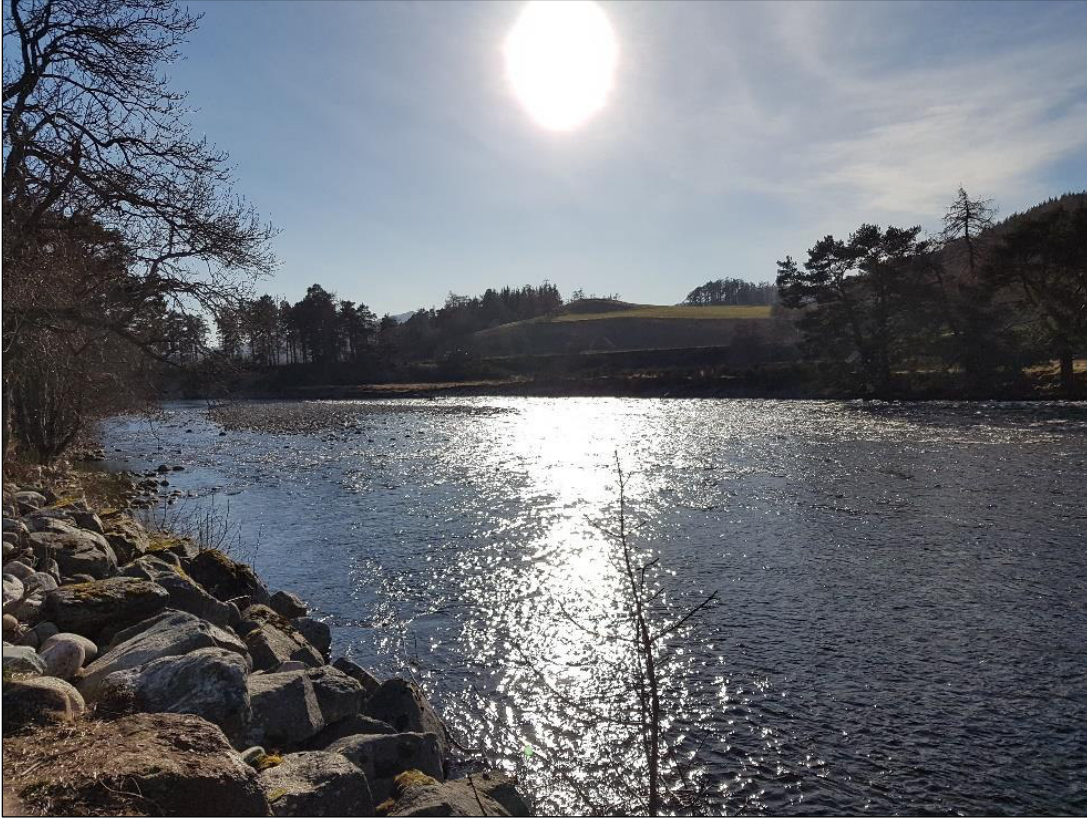
FIGURE 5 – FLOOD DEFENCES LEFT BANK
